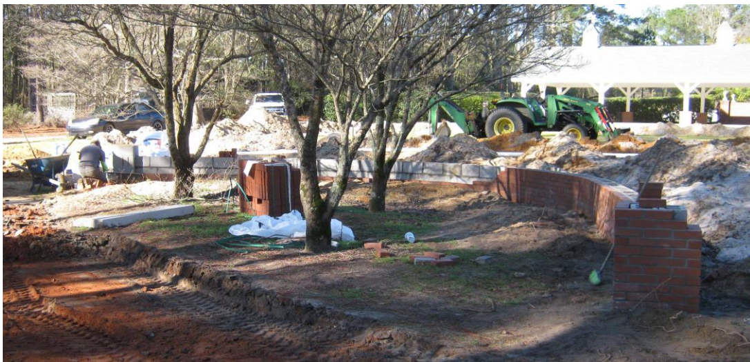
Master Mason Helbreth at Work on the Brick Walls
